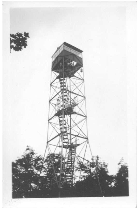
The Valley Forge Fire Tower (circa 1932) The tower was dismantled about 1939 due to safety considerations.
